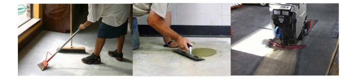
Fill any holes and nail in protruding nails in your floor. This should be completed at this stage so you end up with the optimal fresh clean flat surface to begin your job.
